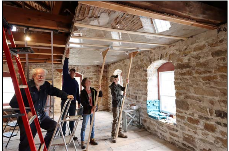
Installing Plexiglas. Art Shaw (left) with Moel Benoit, John Cairncross and Carter Perkins.
