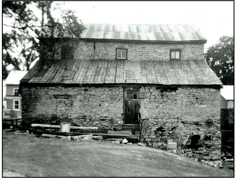
This mid-1960s photo of the west side of the mill shows the sorry state of the turbine hall and the rusting galvanized steel roof of the mill. The sawmill, which was attached to the mill, has been mostly removed by this time, just a bit of the flooring remained.
