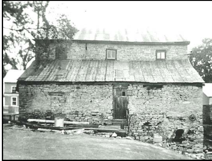
Turbine Shed Roof
